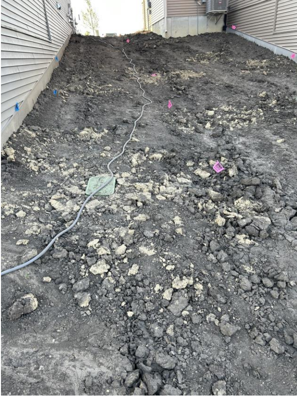
Figure 2. Clay exposed due to irrigation installation
